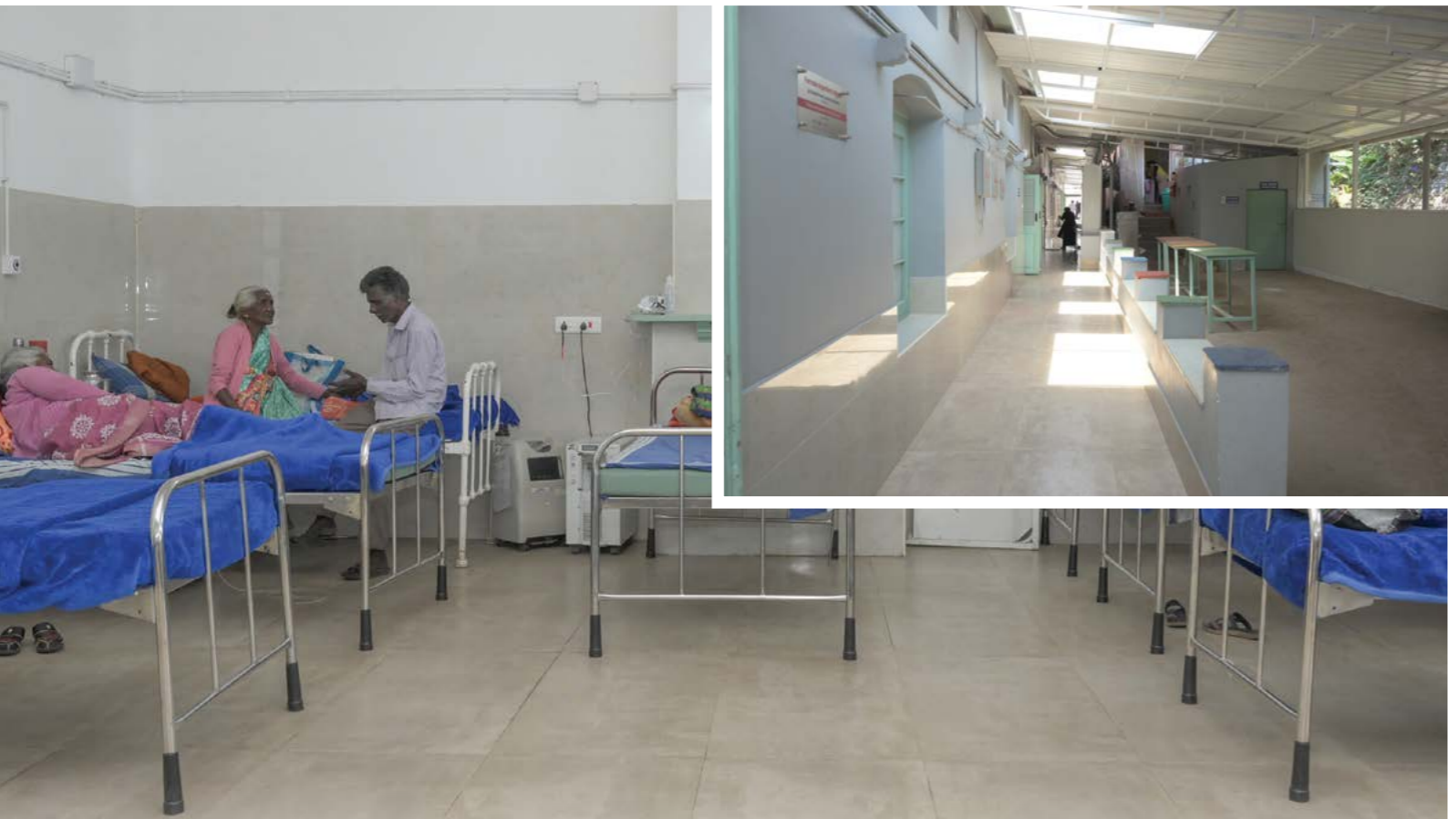
Upgraded infrastructure with skid-proof flooring, improved lighting, dedicated spaces for caregivers, clean beds, and protective mesh installations to enhance patient comfort and security. Lawley Hospital is now a place where care feels visible in every corner.
